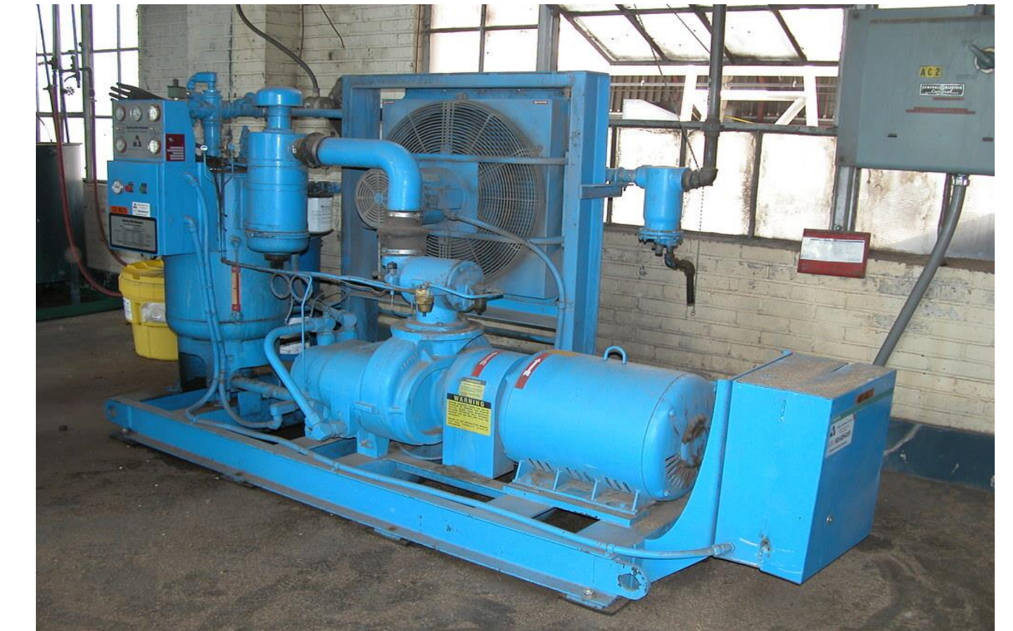
An oil injected rotary screw air compressor.
